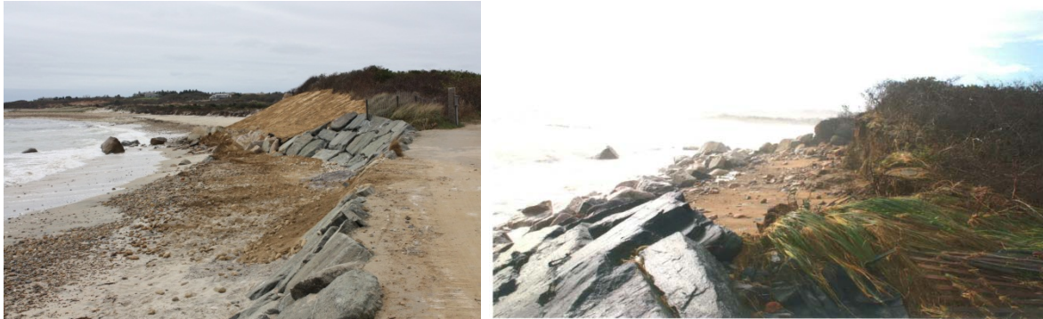
Figure 3. The “soft-solution” before Hurricane Sandy on the left and after Hurricane Sandy on the right.
