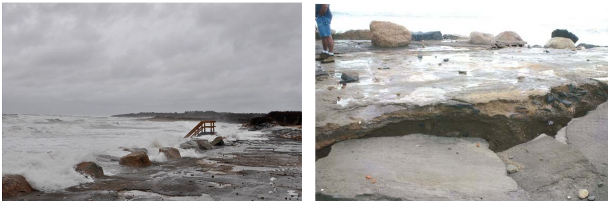
Figure 2. Town Beach Parking Lot during Hurricane Sandy.
